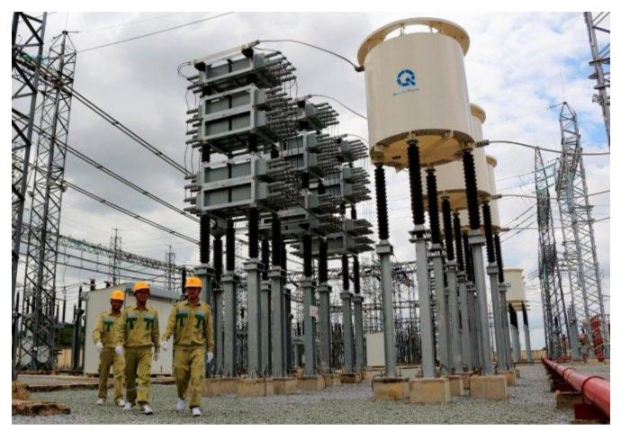
Capacitor banks are electrical devices designed to improve power factor and voltage stability in electrical power systems. They consist of a series of capacitors connected in parallel with the electrical distribution system. Capacitor banks are commonly used in industrial, commercial, and utility settings to compensate for reactive power and enhance overall system efficiency.
